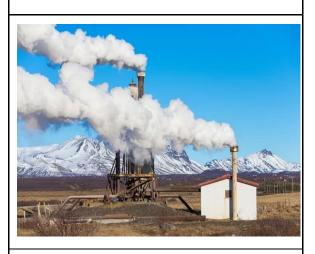
Source: Daniel Allen Description: Water is pumped beneath the ground to hot areas and the steam from the water drives turbines to produce electricity
